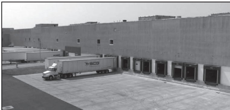
York Business Center EGL dock fit-out
